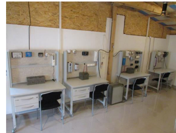
PV Lab at Mithradham for practical training (2016)
